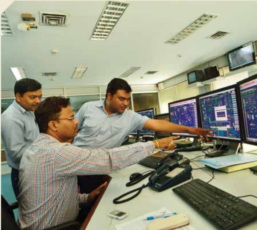
▲ Central control room
