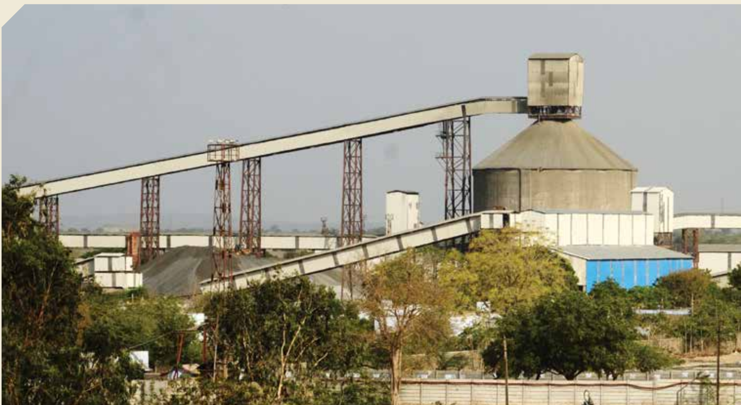
Full View of the New Grinding Unit at Morak
